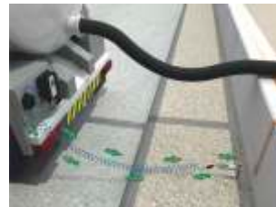
Continuous Ground Loop Monitoring check
